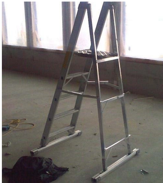
Figure 2. An A-ladder whose overall stability is secured with, for example, a stabiliser may also be used when an employee stands on its work platform at a height of 1 to 2 metres (the minimum stabiliser bar length is 90 cm).
