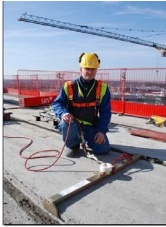
Figure 5. Appropriate fall protection must always be worn when working at height, for example, on a roof.
