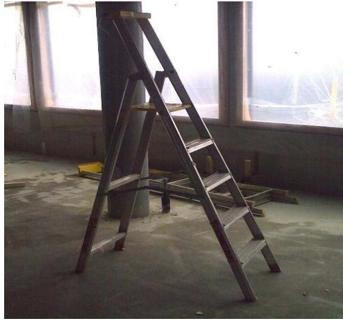
Figure 1. This may only be used when the employee stands on it at a height of less than 1 metre. Recommendation: A-ladders without stabilisers should not be used!
