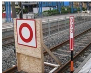
Figure 2. STOP board. This board must always be used when a track is closed for traffic for the duration of track work.
