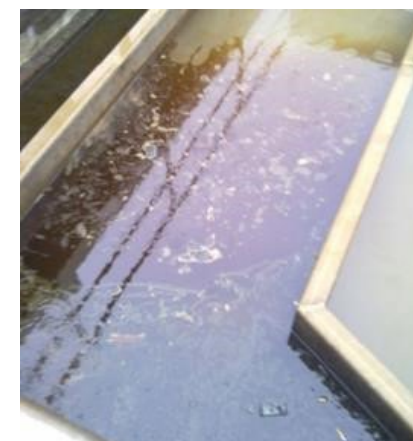
The sedimentation basins at the wastewater plant are equipped with oil troughs.
